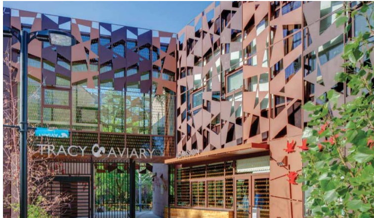
Figure 3: An architecture which incorporates a mix of decorative grilles and fritted window patterns to reduce bird strikes (Photo: Alan Blakely, 2015) 1
