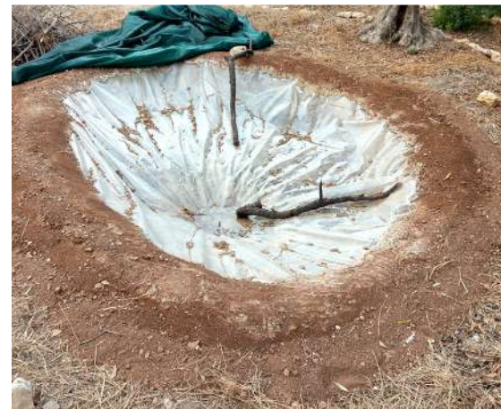
Freshwater pond in final stages of construction
