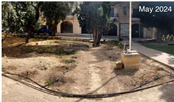
Entrance area a year apart: artificial turf has been removed, the soil ploughed up and planted with shrubs, which are watered by drip irrigation; note also nature trail dug in preparation for aggregate layer.
