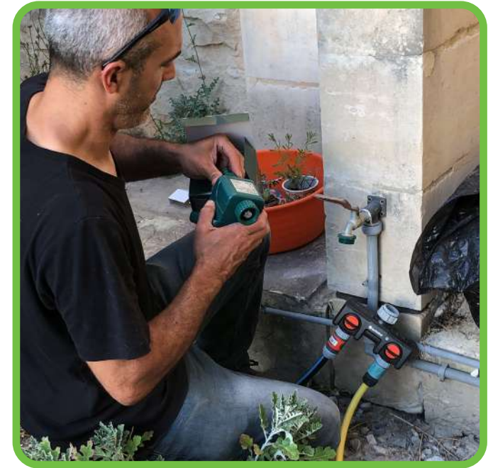
A battery-operated timer is an important component of a drip irrigation system, so you can control how often and at what time your plants are watered.
