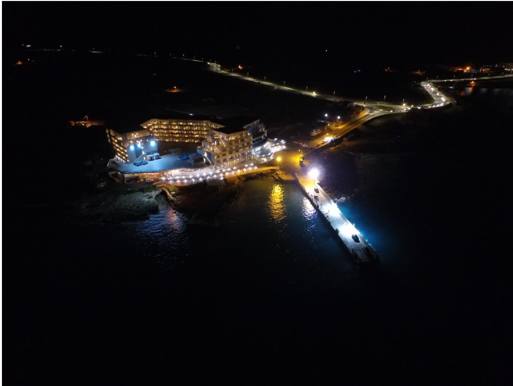
Figure 1: Aerial view at night of Marfa jetty showing incompatible and insensitive lighting at night of the area
