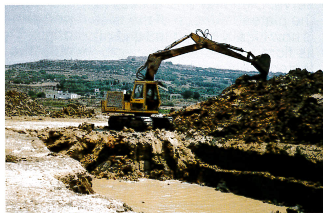
Heavy machinery at Is-Simar creating ditches, pools and islands.
