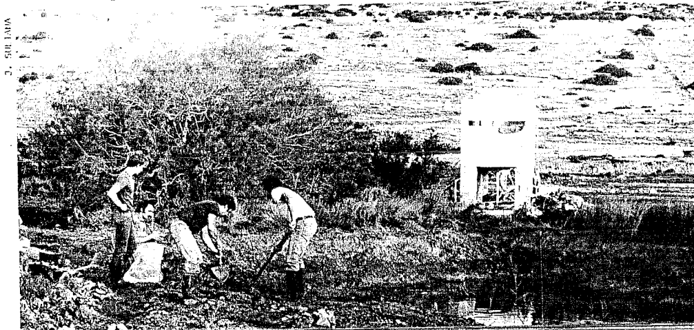
After the machines left the area MOS members have been maintaining the momentum of work by hand tools - planting trees and shrubs, constructing islands and fencing the area.
